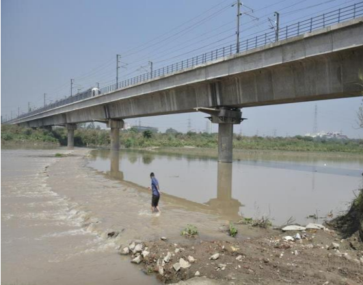
Figure 4. Metro bridge along Yamuna river bed
