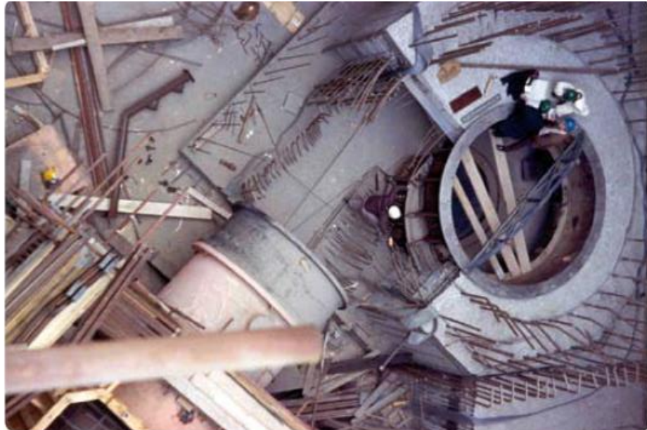
Concrete volute pump under construction
