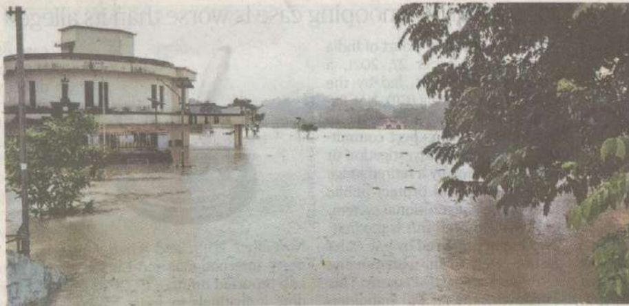
No trace: A flooded municipal stadium in Pathanamthitta district on Monday. • LEJU KAMAL
